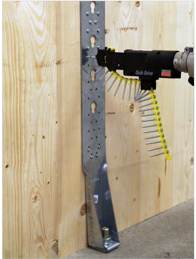
Quik Drive collated CSA screws fastening HTT31 holdown in CLT wall to concrete slab installation.
